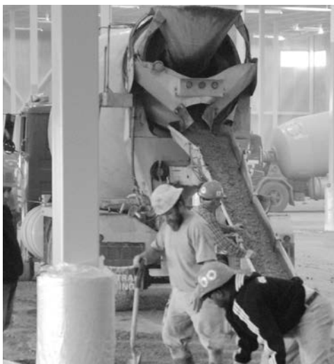
Used to carry fresh concrete from the batch plant to the jobsite
