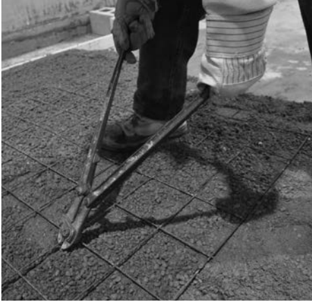
Used to cut wire mesh
