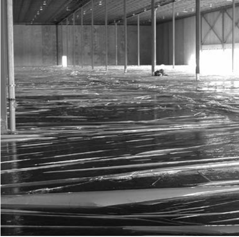
Used to harden the concrete surface. Wet curing covers such as polyethylene sheets are laid over new concrete
