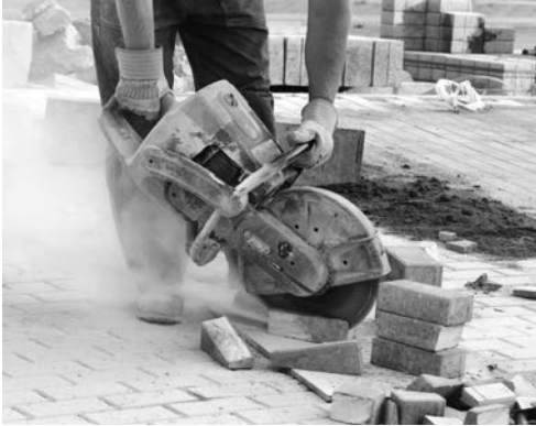
Used to cut contraction joints and rebar materials
