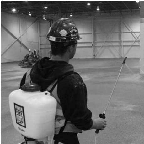
Used to apply form oil, sealers, and evaporation reducers
