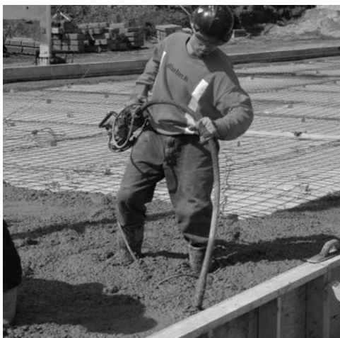
Used to consolidate concrete around reinforcing steel and to remove air pockets
