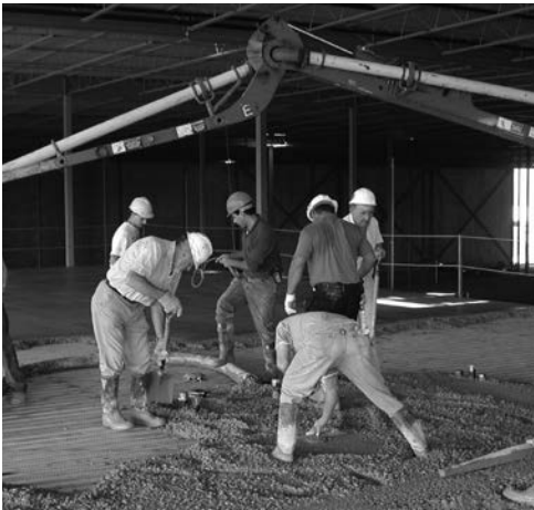
Used to carry fresh concrete from the concrete truck to the point of deposit
