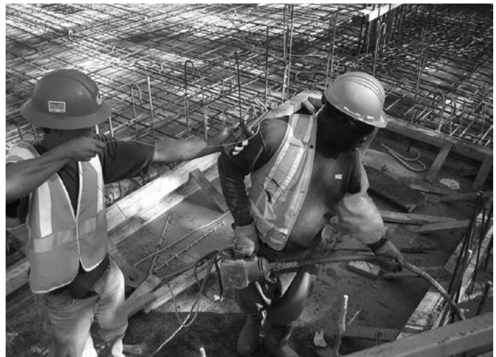
Figure 6-11: Testing Noise Levels in the Workplace
