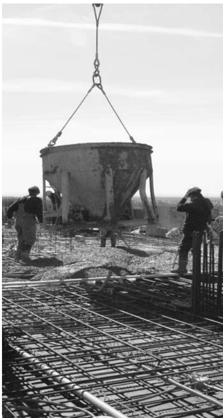
Used to carry fresh concrete from the concrete truck to the point of deposit
