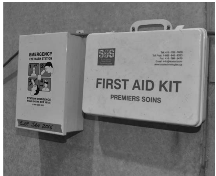
Figure 4-3: First Aid Box and Eye Wash Station
