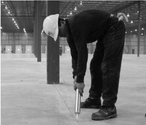
Used to fill joints in the floor
