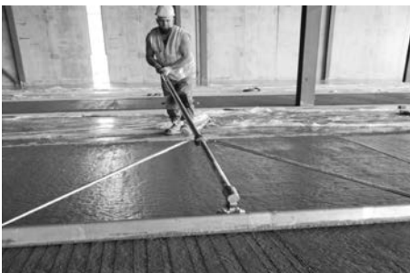
Used to improve flatness of surface
