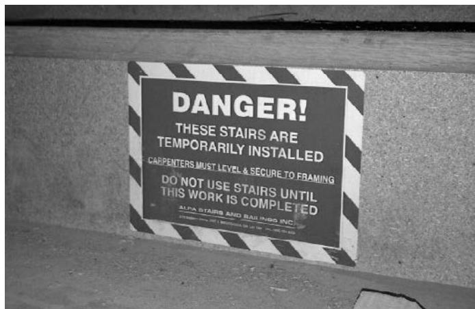
Figure 9-13: Warning sign on temporary stairs
