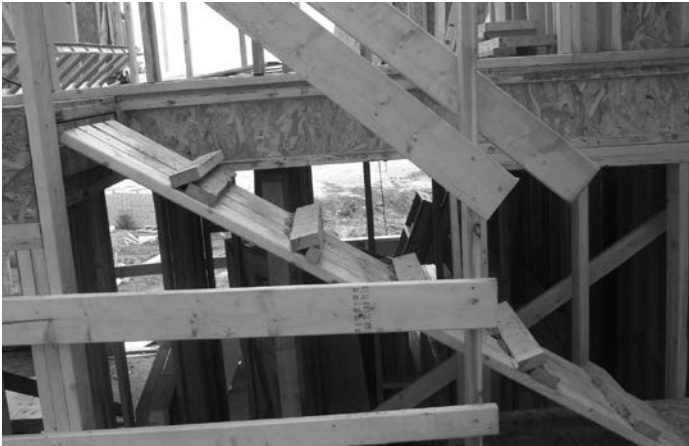
Figure 9-9 Ramp is not strong enough or not at the proper slope to be used as a stairway.
